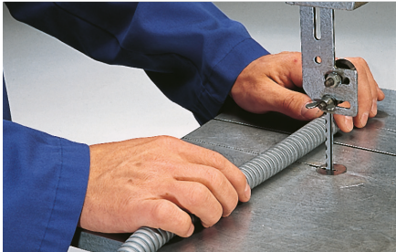
Position conduit at right angles to band saw
