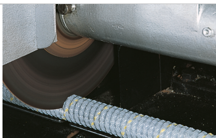
Cut through the conduit with low pressure clean ends
