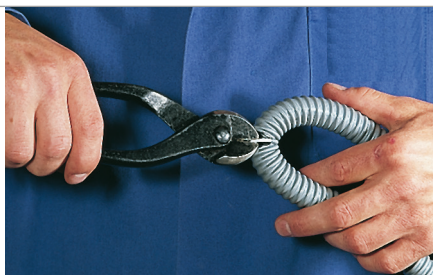
Bend the conduit and cut through the helix
