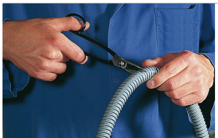
Cut through the plastic sheathing
