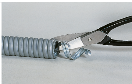
Cut off with snips. Uncoil one or two segments and cut off. Press in the ends and snip off the protruding corners.
