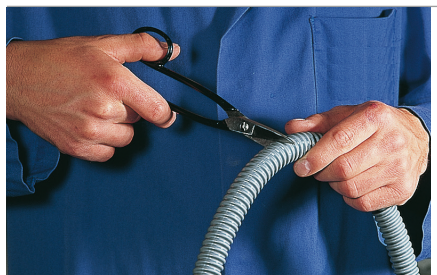
Cut through the plastic sheathing
