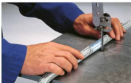
Bind conduit with metal adhesive tape at the cutting position 2 or 3 times
